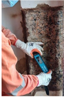
Figure 1. Measurement of surface resistivity
