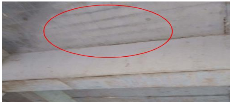
Figure 9. Slab bottom reinforcements visible
