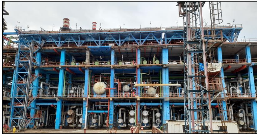
Figure 2. Image after rehabilitation & retrofitting
