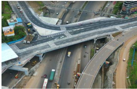
Figure 1. Chandani chowk Bridge, Pune
