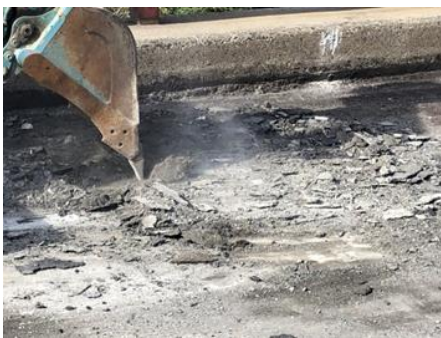
Figure 1. Cutting of base layer asphalt concrete
