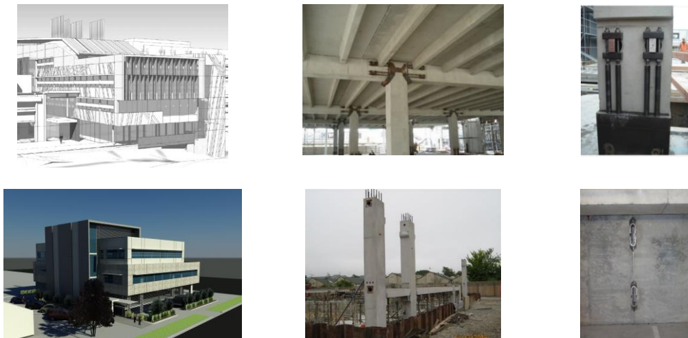
Figure 4. Top: First multi-storey PRESSS buildings in NZ. Unbonded Post-Tensioned (PT) frames with external Plug&Play dissipaters and PT walls coupled with steel beams (Struct. Engineers: Dunning Thornton Consultants; Cattanach and Pampanin, 2008). Bottom: Southern Cross Hospital Endoscopy Building, Christchurch. PT frames with internal (top-only) mild steel and PT walls coupled with UFPs (Struct. Engin.: Structex Metro, Pampanin et al., 2011).
