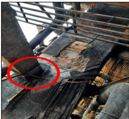
Figure 5. Carbon fiber wrapping burned
