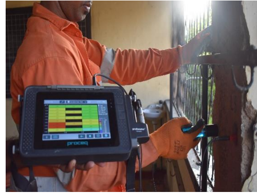
Figure 2. Half-cell potential testing on column location
