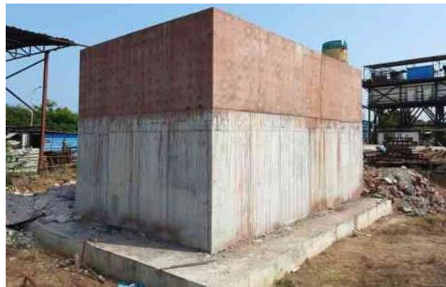
Figure 2. Completed heavy density slab
