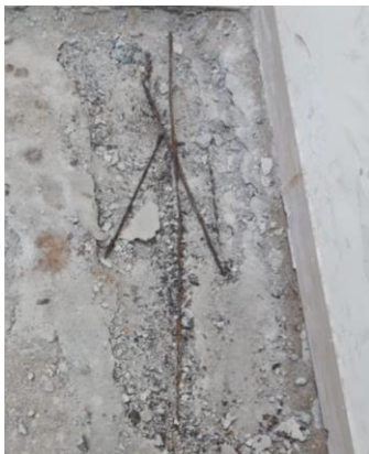
Figure 2. Corroded Reinforcement
