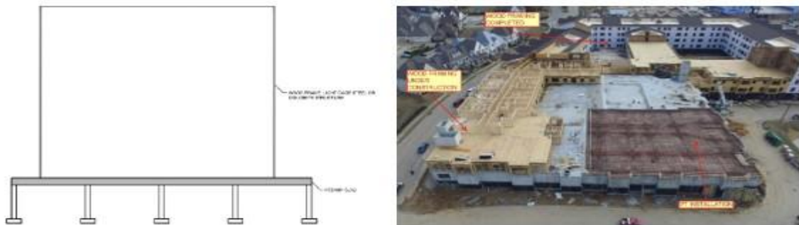
Figure 4. Use of Podium slab to support superstructure made of different materials (wood, steel, precast, CIP concrete)
