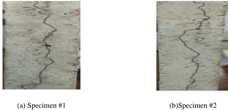
Figure 4. Crack Pattern observed on surface of Mortar Specimens of D type aggregate.
